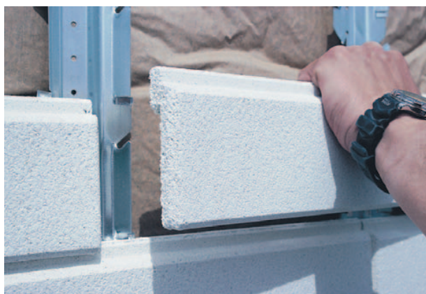
Marmoroc under montering
